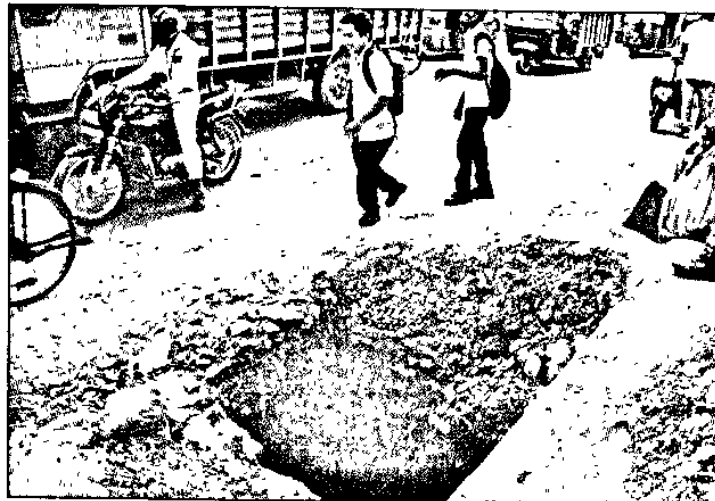
■ The uncovered drains on Aurobindo Marg, near IIT gate, could lead to avoidable accidents.
